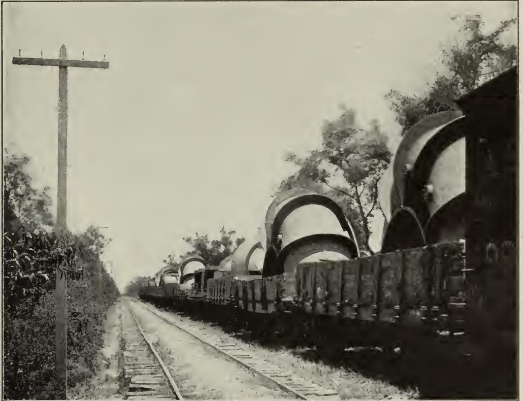
TRAIN LOAD OF PUMPS FOR PUMPING STATION NO. 7.
